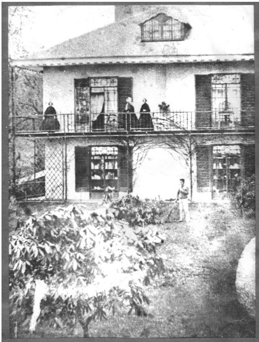
Claremont, about 1856–64 by the dress: three ladies on the balcony, and a man in the garden.
